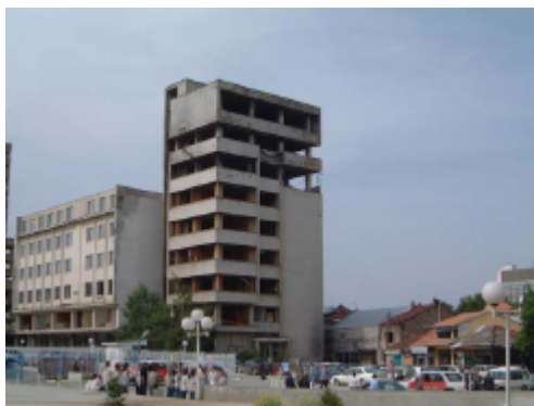
EAR tower in Pristina/Kosovo before refurbishment
